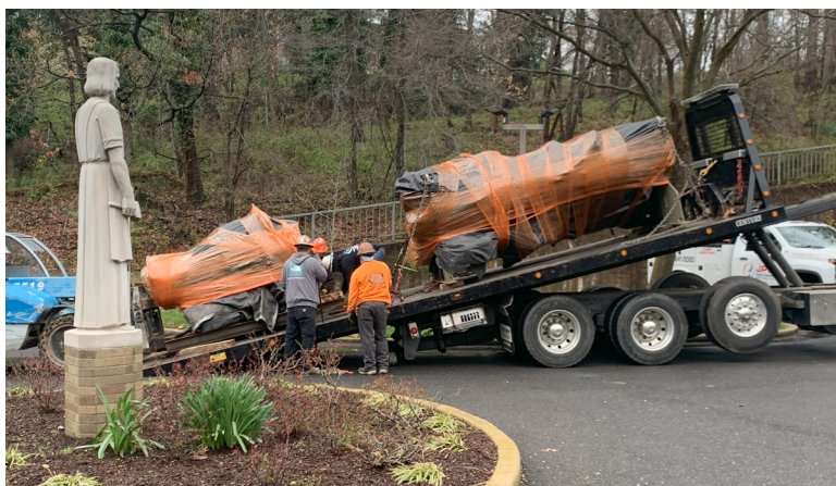
Sr. Joseph with the broken 300-ton chiller, that is wrapped in chains for removal. The plan to hoist it out whole was thwarted by its size and the presence of a giant blue pipe. “Instead, it had to be cut apart to be removed,” said Sr. Joseph emphasizing the massive scale of the operation. Above right: Under the watchful eyes of our patron saint, St. Joseph, it took several hours to carefully unload the new chiller.
